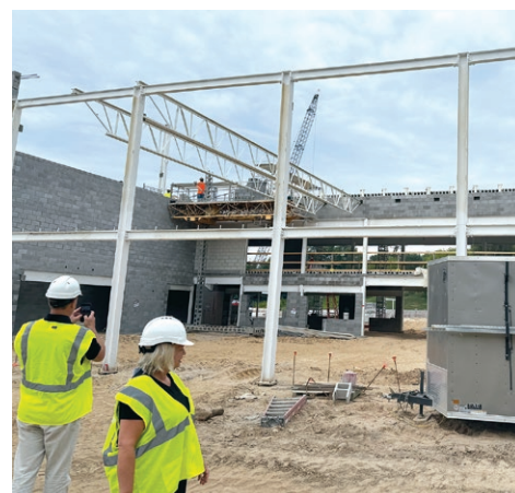
Construction is underway at the new aquatic center site.
