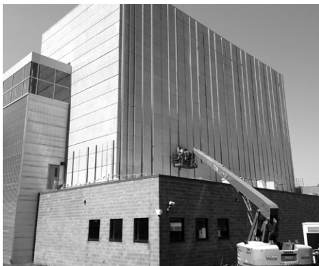
Renovations on several district buildings are underway this summer! The upper photo shows interior work progressing on Eastern's gymnasium addition. The lower photo reveals the exterior work on the Fine Arts Center.
