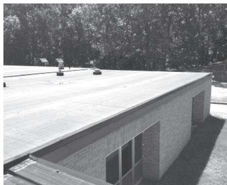
Thornapple Elementary School received a new roof, including new steel decking, edge metal, and flashings.
