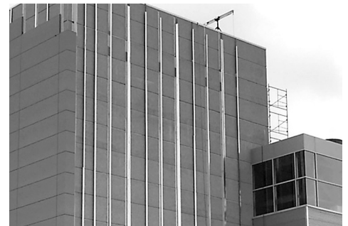
Construction workers install new flashing on all sides of the building and repair the fly loft above the stage at the Fine Arts Center.
