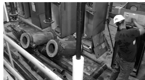
Last summer, four FHPS schools installed new boiler systems as part of the district's bond projects.
